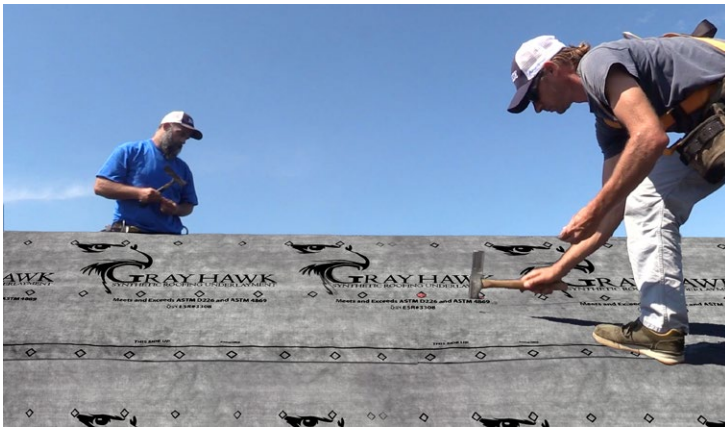
Nailing Pattern For Gray Hawk In Normal Conditions Using Regular Roofing Nails or Cap Nails
